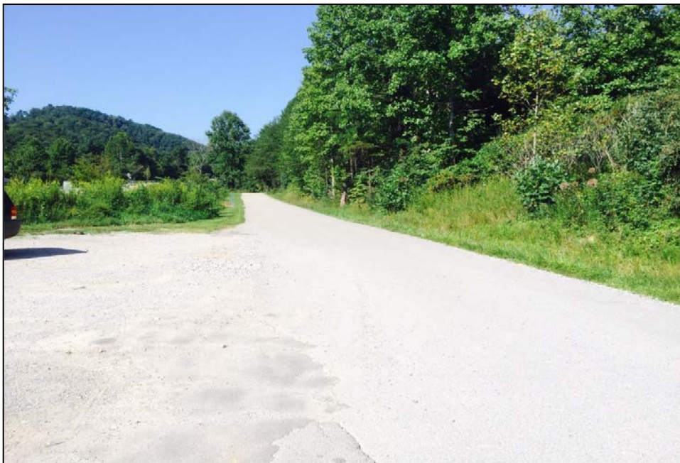
Intersection of Urban Creek Rd and HRP, looking southwest down Urban Creek Road
