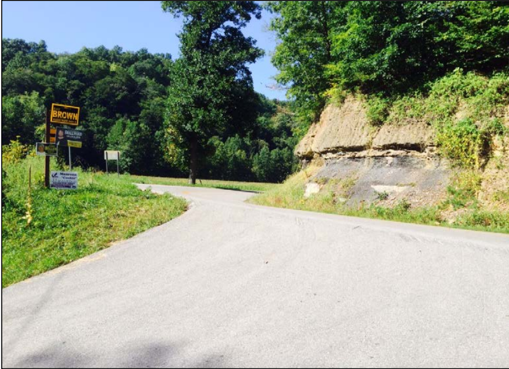
Intersection of Urban Creek Rd. and KY 687, standing on Urban Creek Rd. looking west on KY 687
