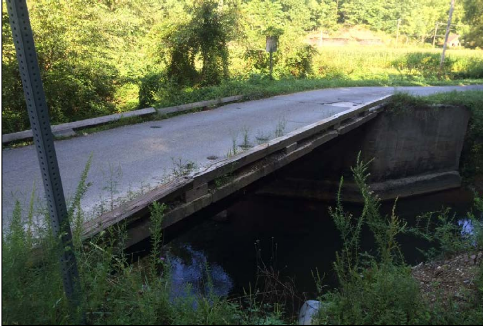
Bridge No. 026C00071N, east side of bridge
