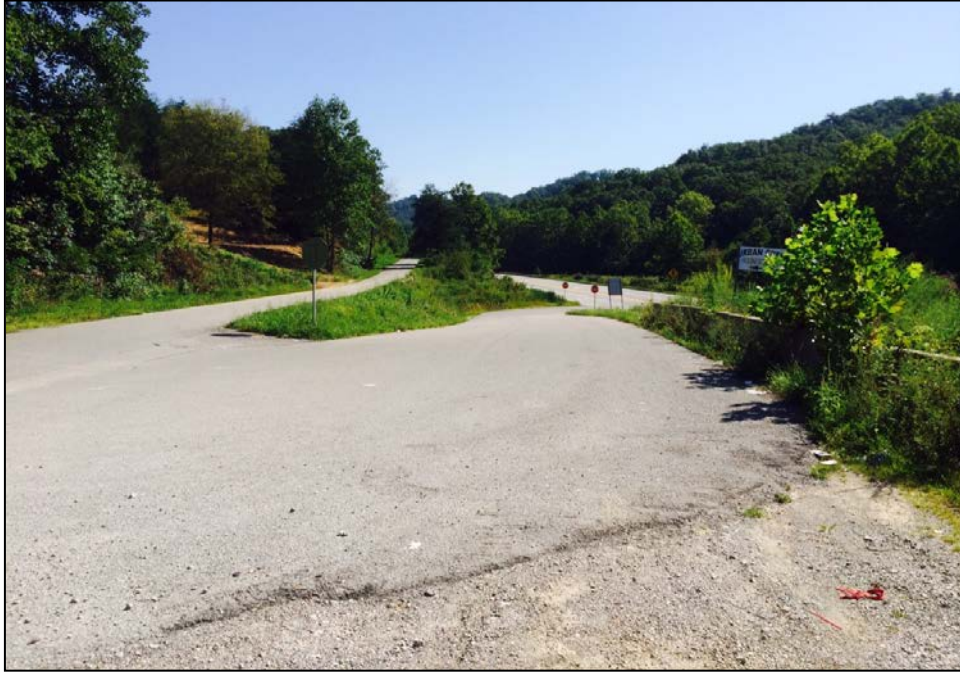
Intersection of Urban Creek Rd (left) and Hal Rogers Parkway (right), looking northeast
