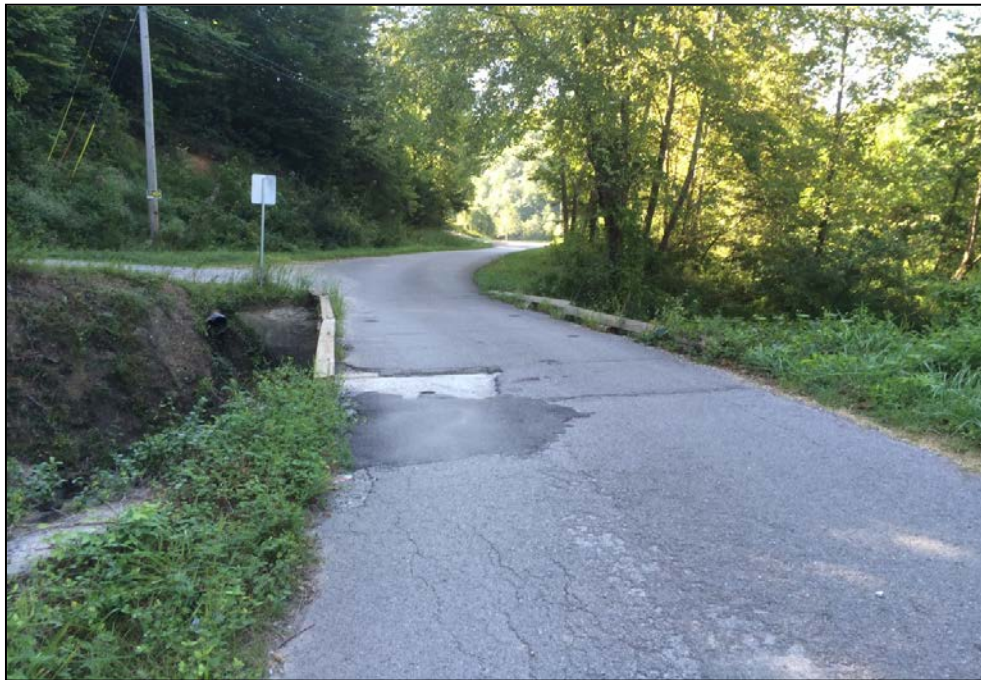
Bridge No. 026C00071N, looking south east across bridge
